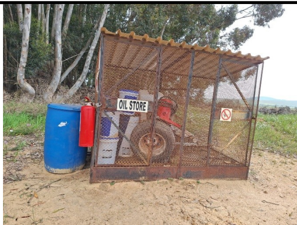
DIESEL TANK – DRIP TRAY BE PLACED UNDERNEATH
